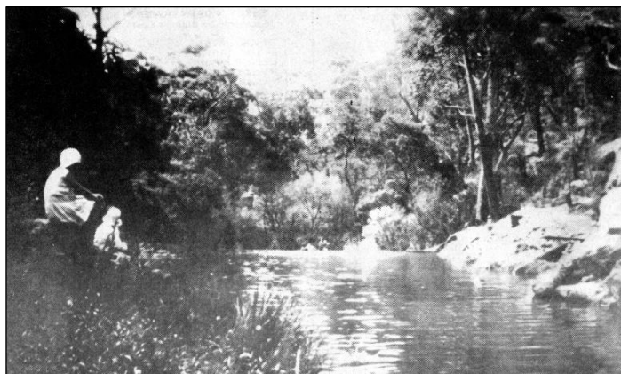
An early view of the dam, this photo was obtained by locals from the Railways Dept in 1928.
